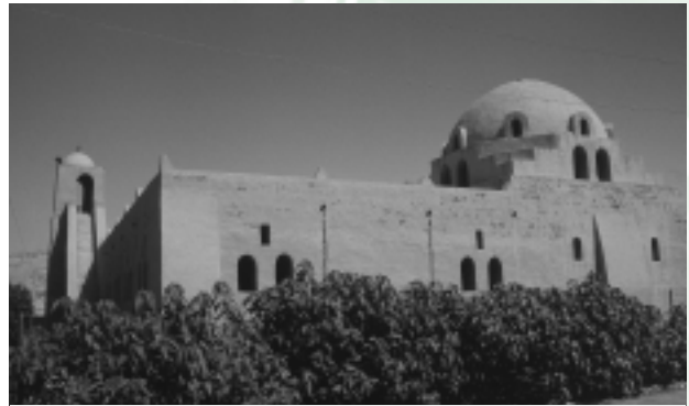
Fig. 14: New Gourni mosque, Luxor, Egypt. Designed by Hassan Fathy and built with sun dried earth blocks.
